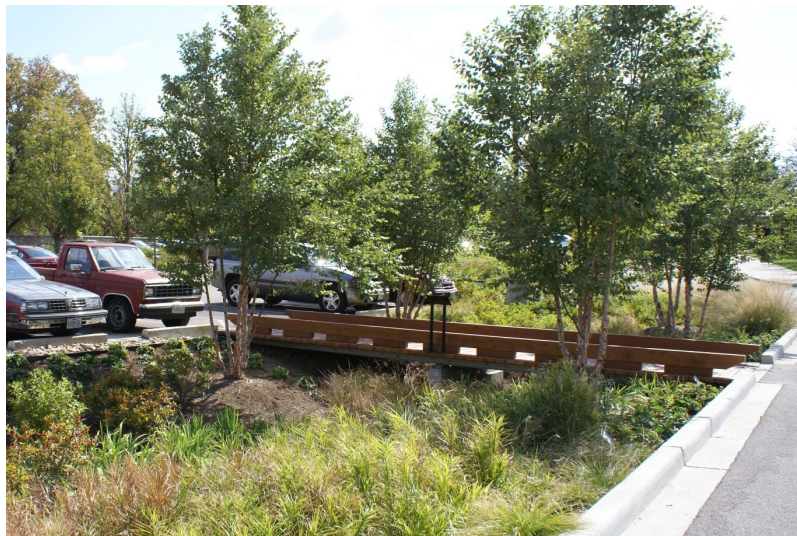
Parking Lot Drainage Enhancements
