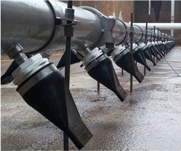
Figure 5-14 Proposed Duck Bill Digester Diffusers
