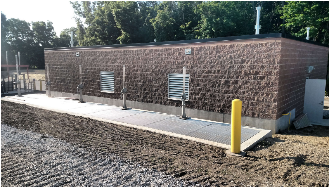
Figure 5-7 Filter Influent and Bypass Gates
