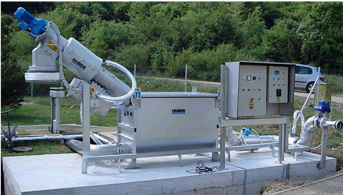
Figure 5-6 Proposed Septage Receiving Station
