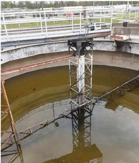
Figure 5-2 Existing Secondary Clarifier No. 1
