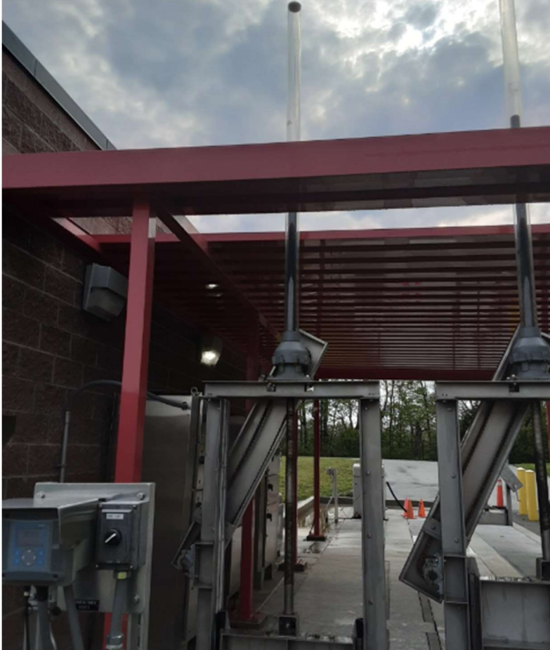
Figure 5-4 Existing UV Canopy
