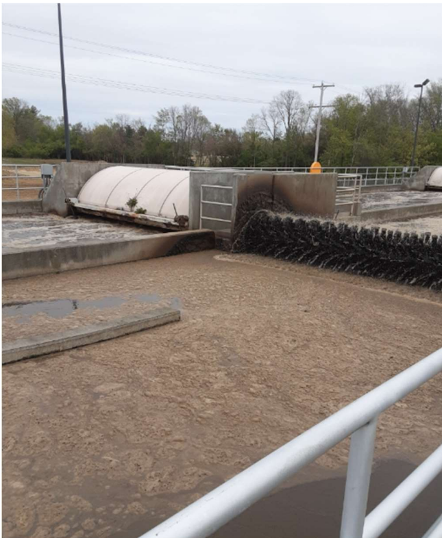
Figure 5-1 Existing Oxidation Ditch 3
