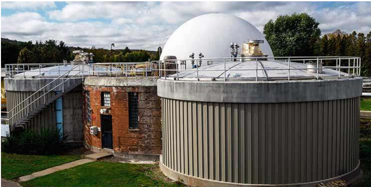
Figure 4-15 Anaerobic Digester Example
