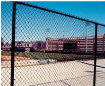
Basis: Ameristar Permacoat Chain-Link Fence or similar product. Finish: Black or green vinyl coated Features: Only to be used for low visibility areas that require security.
