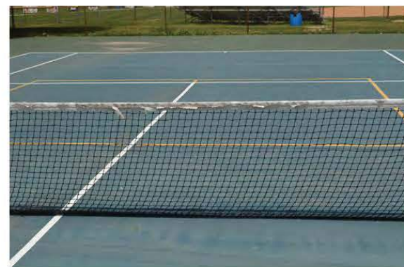
Tennis Courts / Wear & Tear
