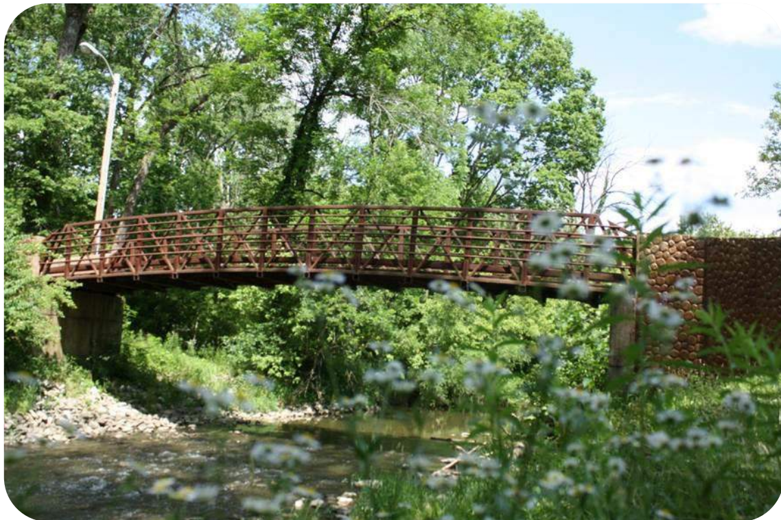
Bridge at Arbuckle Acres Park
