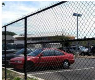
Basis: Ameristar Permacoat Chain-Link Fence or similar product. Finish: Black or green vinyl coated Features: Only to be used for low visibility areas that require security.
