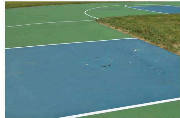
Basketball Courts / Surfacing & Cracking
