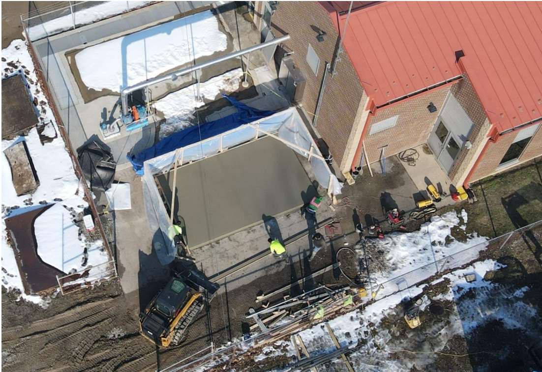
East Plant (main pumping station) – concrete pad for odor control system
